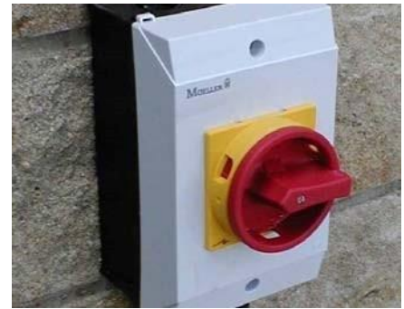
Rotary Isolation Switch
